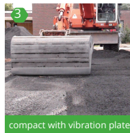
compact with vibration plate
