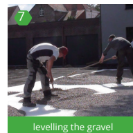
levelling the gravel
